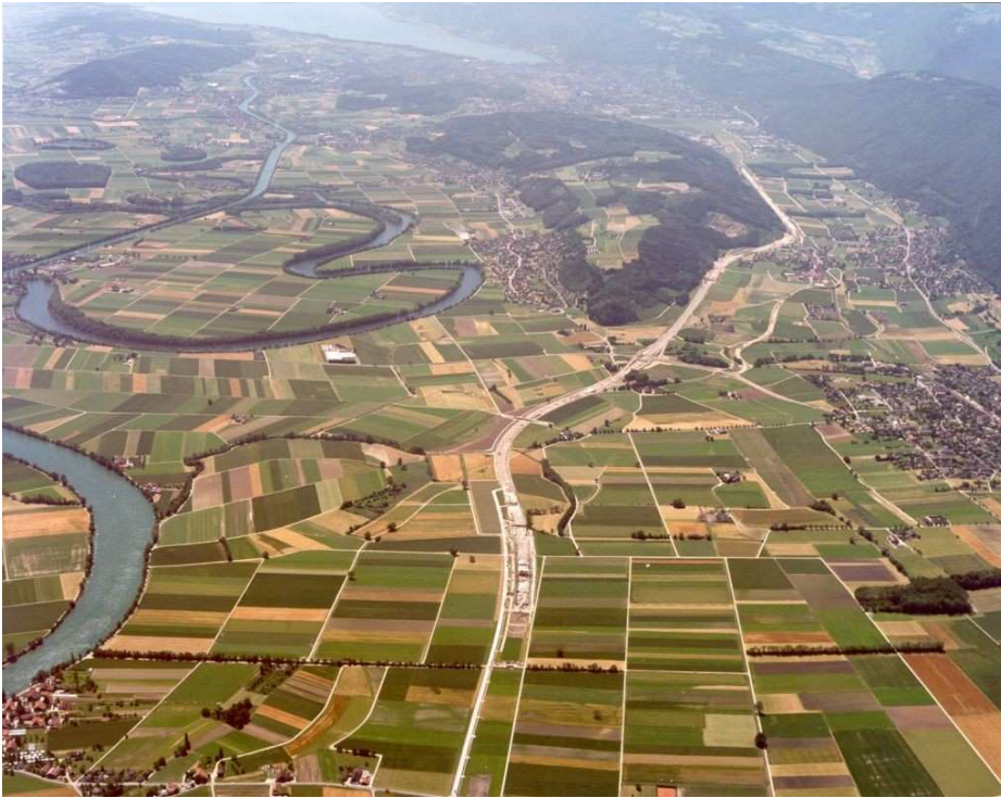
Figure 7: Construction of the covered passage at Grenchen Wyti (FOEN).
